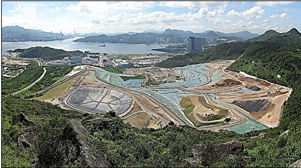
Figure 6.10. South East New Territories Landfill lined with geotextile membrane, Hong Kong
