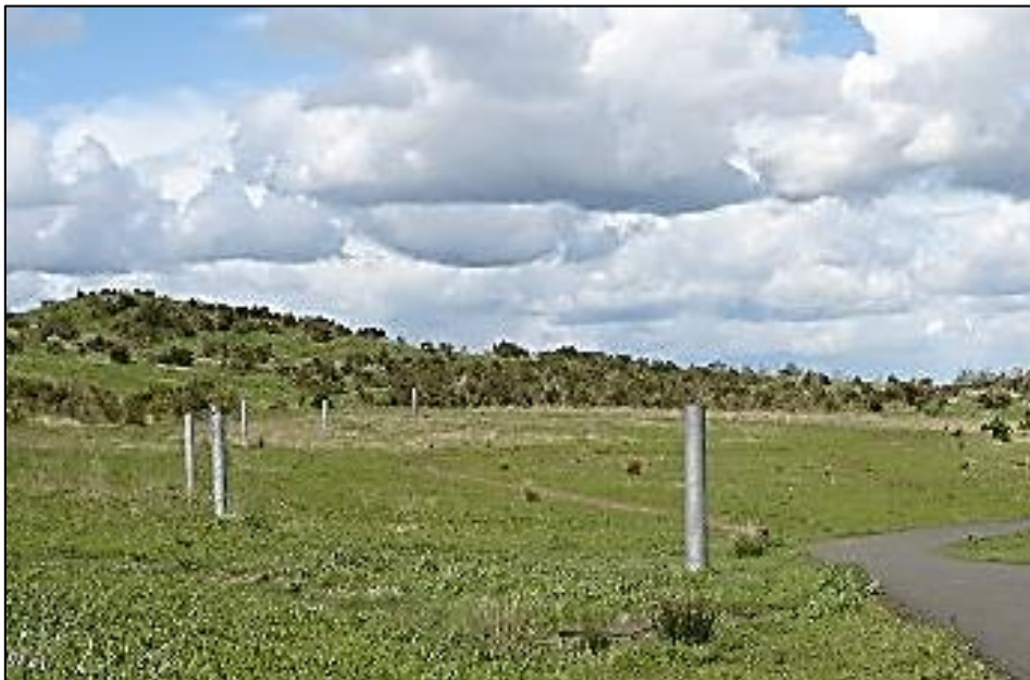
Figure 6.11. Series of methane gas vents on an old landscaped landfill site where oil shale was excavated in the past, Seafield, West Lothian, Scotland
