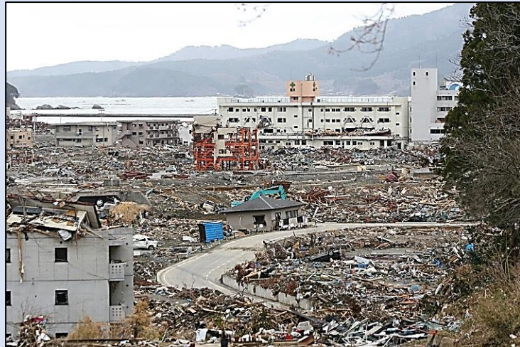
Public hospital in Minamisanriku after the 2011 tsunami
