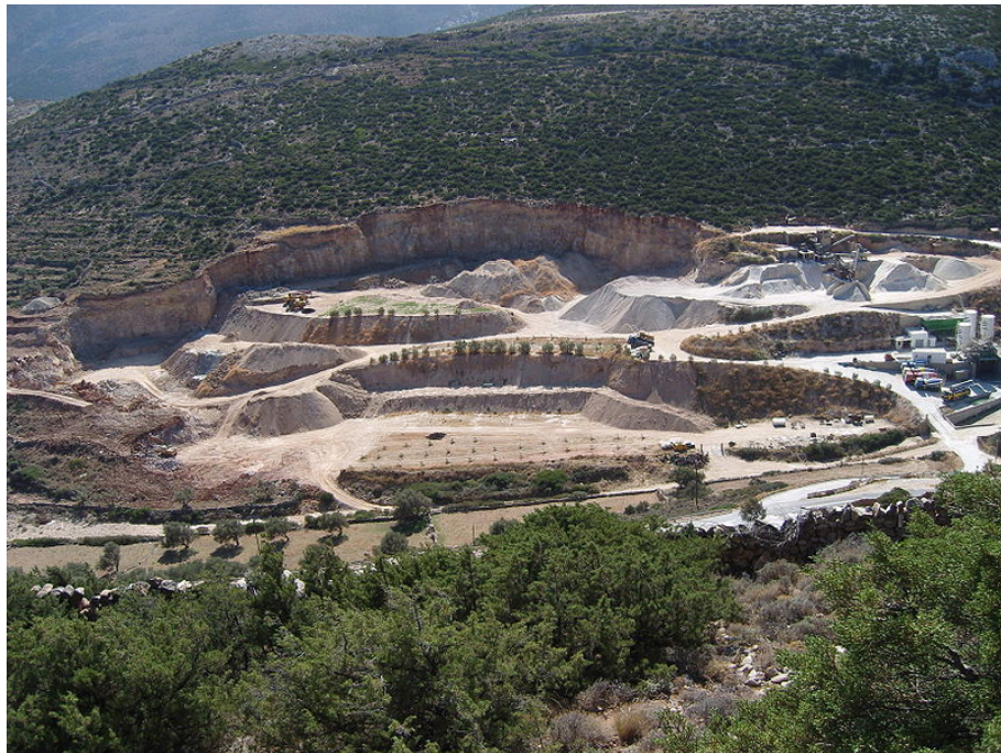
Figure 5.25: A working aggregate-producing quarry on Sifnos, Greece.
