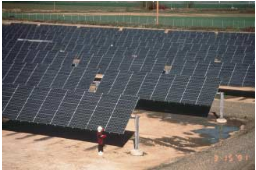
FIGURE 2–19 Solar panels. Davis California Pacific Gas & Electric PVUSA (Photovoltaic for Utility Scale Applications). Solar panels produce dc which must be converted to ac before being fed into the ac system. This plant is rated at 174 kilowatts. (Courtesy Siemens Solar Industries, Camarillo, California)
