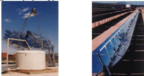
Figure 3: Dish system for concentration sunlight, Parabolic trough system.
