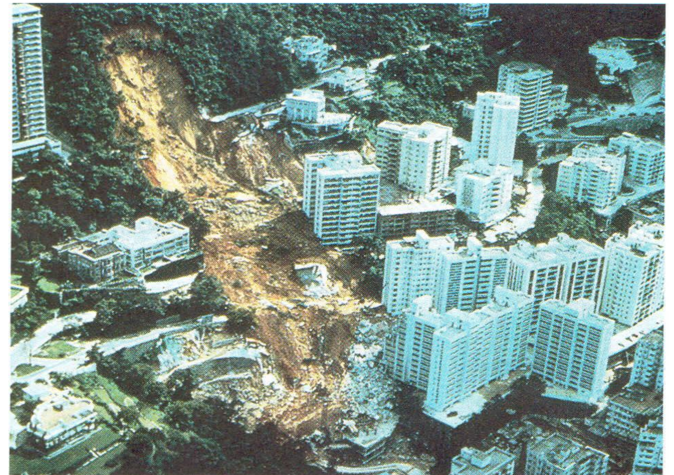
Excavation in hill slope
