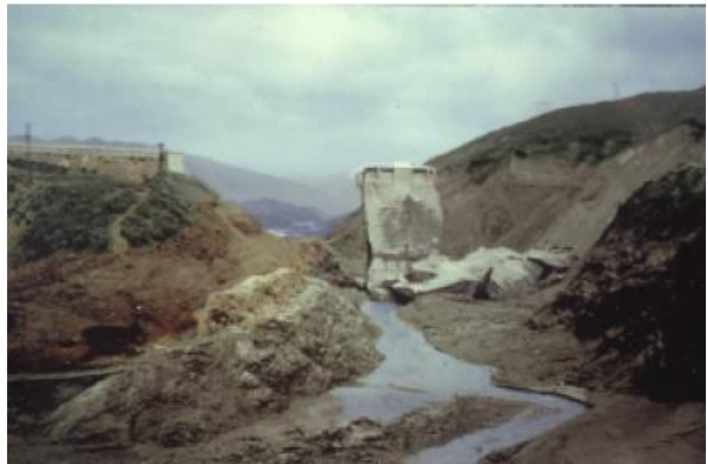
After failure with the 'Tombstone' in the center
