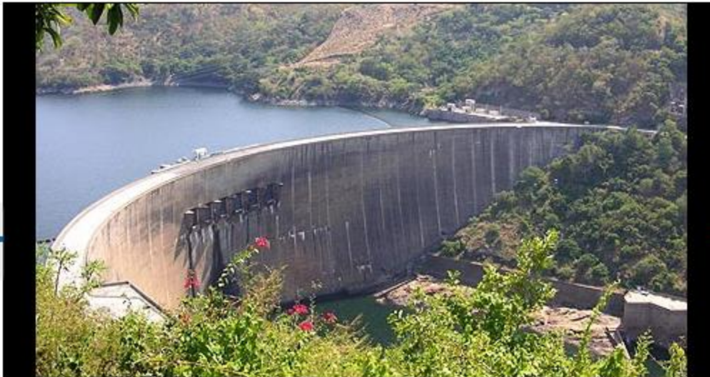
Kariba Dam on the Zambezi River.
