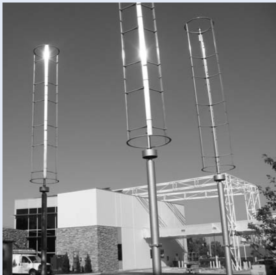
Windspire Turbines. (Picture Courtesy of Windspire Energy.)
