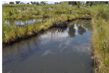
Poor pond construction
