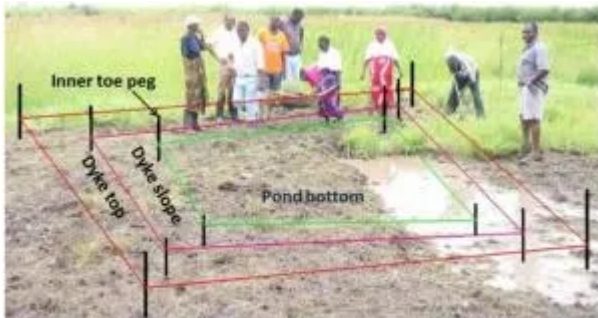
A site pegged ready for digging and filling
