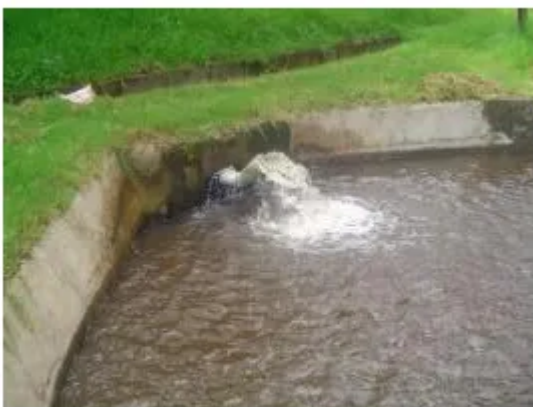
Water inlet for a trout raceway
