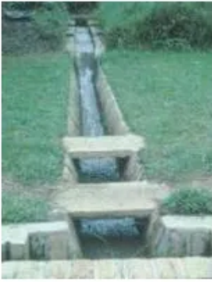
An open water supply canal lined with concrete slabs.
