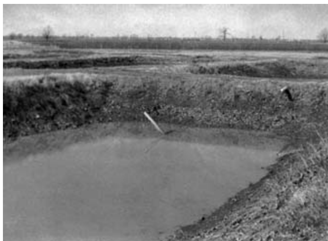
Fig. 6.11 Pond with a turn-down pipe drain. (From Stickney, 1979; by permission of John Wiley & Sons Inc.)
