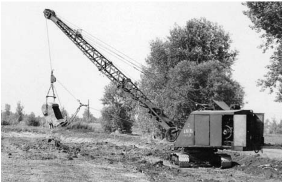
Fig. 6.16 Dragline being used for dike construction. (Courtesy of J. Kovari.)
