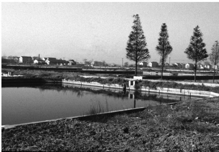
Fig. 2.2. A pond with vertical walls of brick covered with mortar in China.
