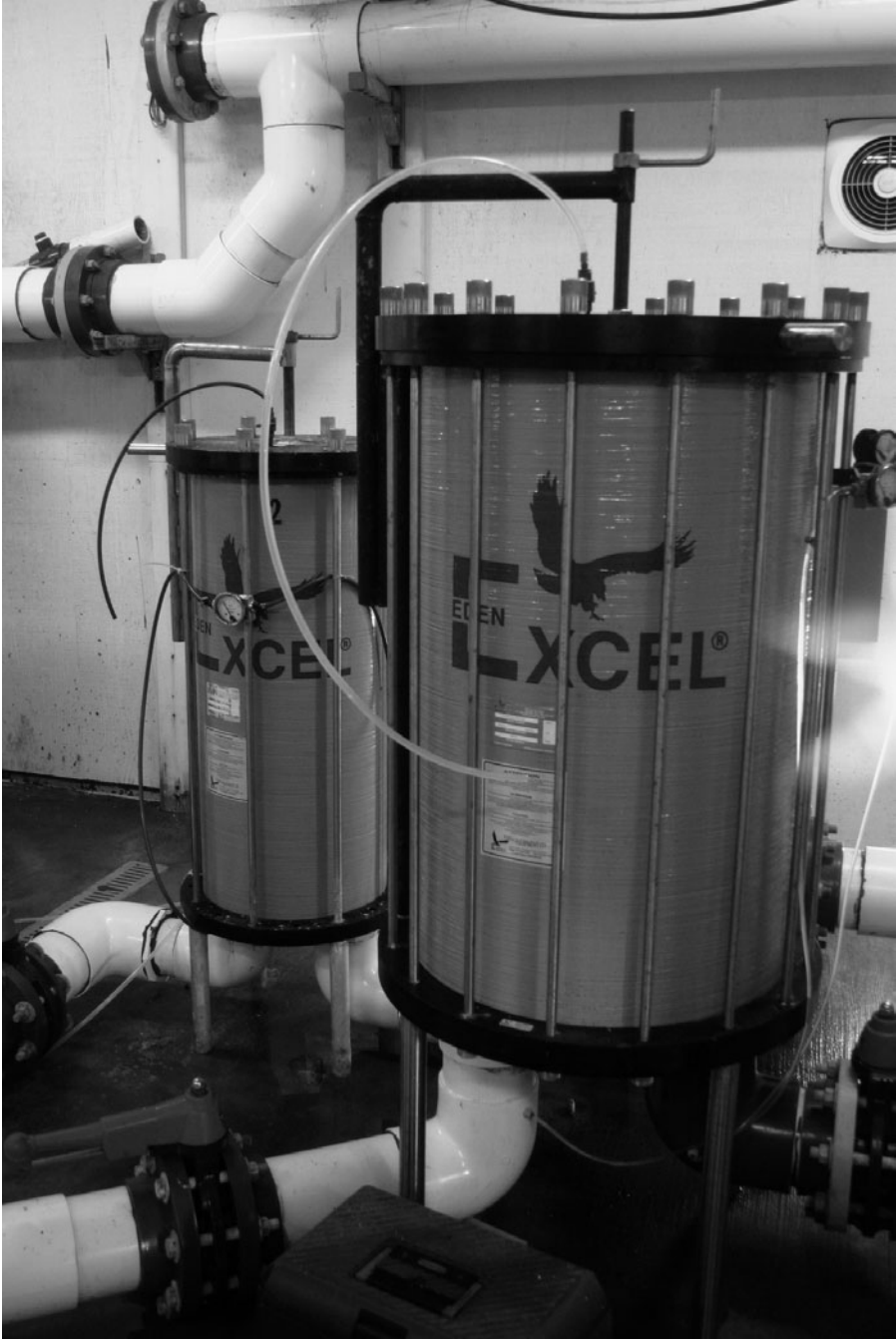
Fig. 2.22. Cartridge filters may be used to remove very fine particulate matter from the water.
