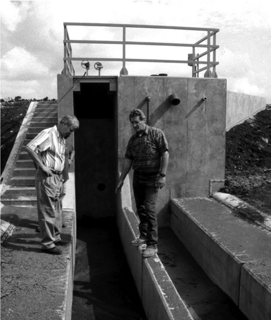
Fig. 2.12. A concrete kettle with access stairway and catch basin in Texas, USA.
