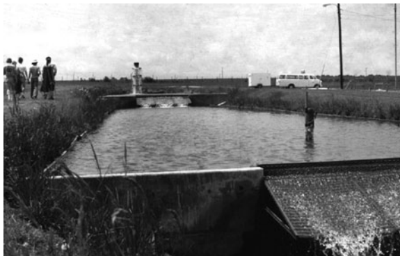
Fig. 2.16. A portion of a series of raceways showing water being aerated as it passes from one to the next. The water entering at the top of the series is aerated at the inflow tower seen in the background.
