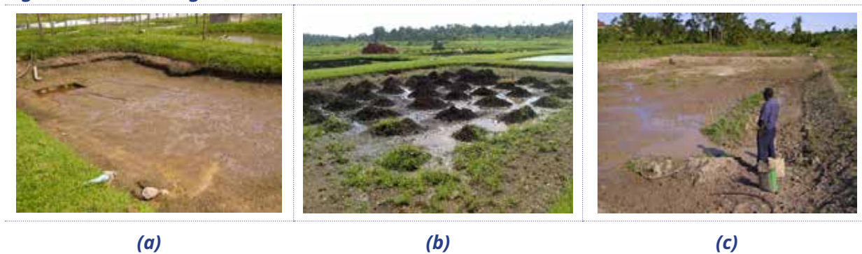
Figure 16: De-silting Ponds
