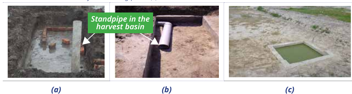
Figure 10: Harvest Basin Inside Pond. When draining pond, standpipe is turned down (b). Harvest basin soon after draining pond (c)
