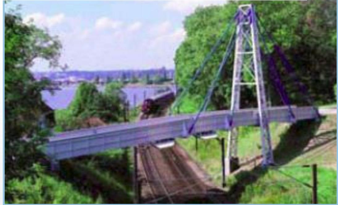
Pedestrian bridge in Denmark, 40 m long (1997)
